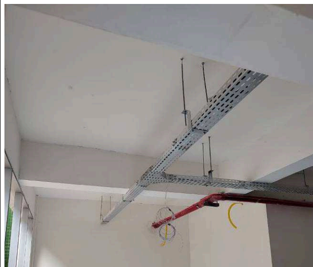
Figura 06: Laje – Hall subsolo.
