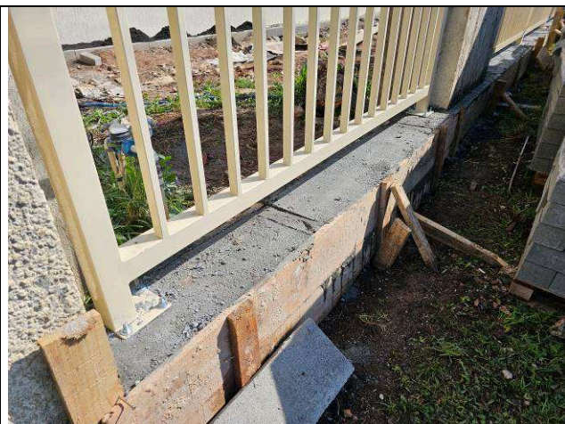
Figura 56: Gradil Frontal – viga baldrame.
