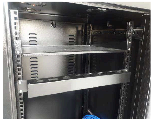
Figura 24E: Rack, bandeja
