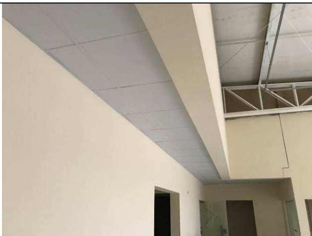
Figura 15C: Forro modular - Hall Central.
