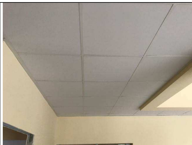
Figura 14C: Forro modular - Hall Central.
