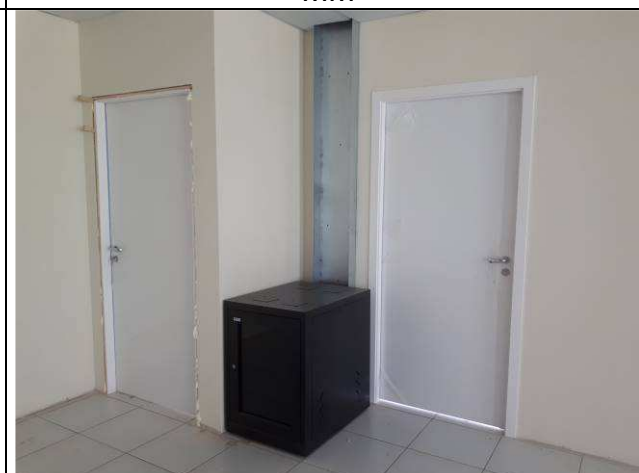
Figura 34E: racks 16U
