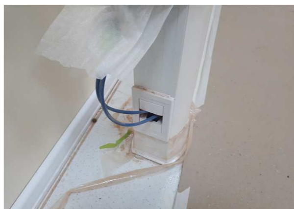
Figura 36E: Patch cord 10m
