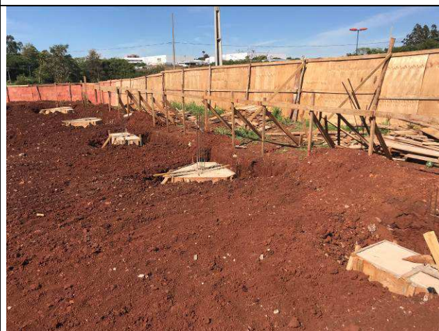
Figura 14C: Blocos concretados - P41, P49, P57, P65, P75.
