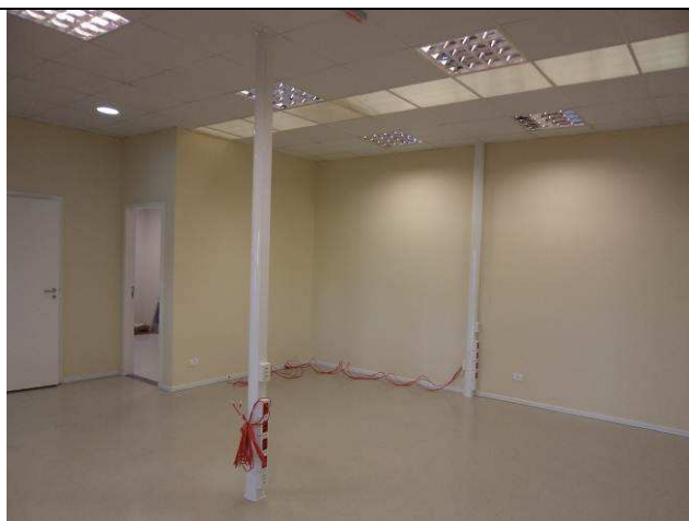
Figura 44E: patch cords.
